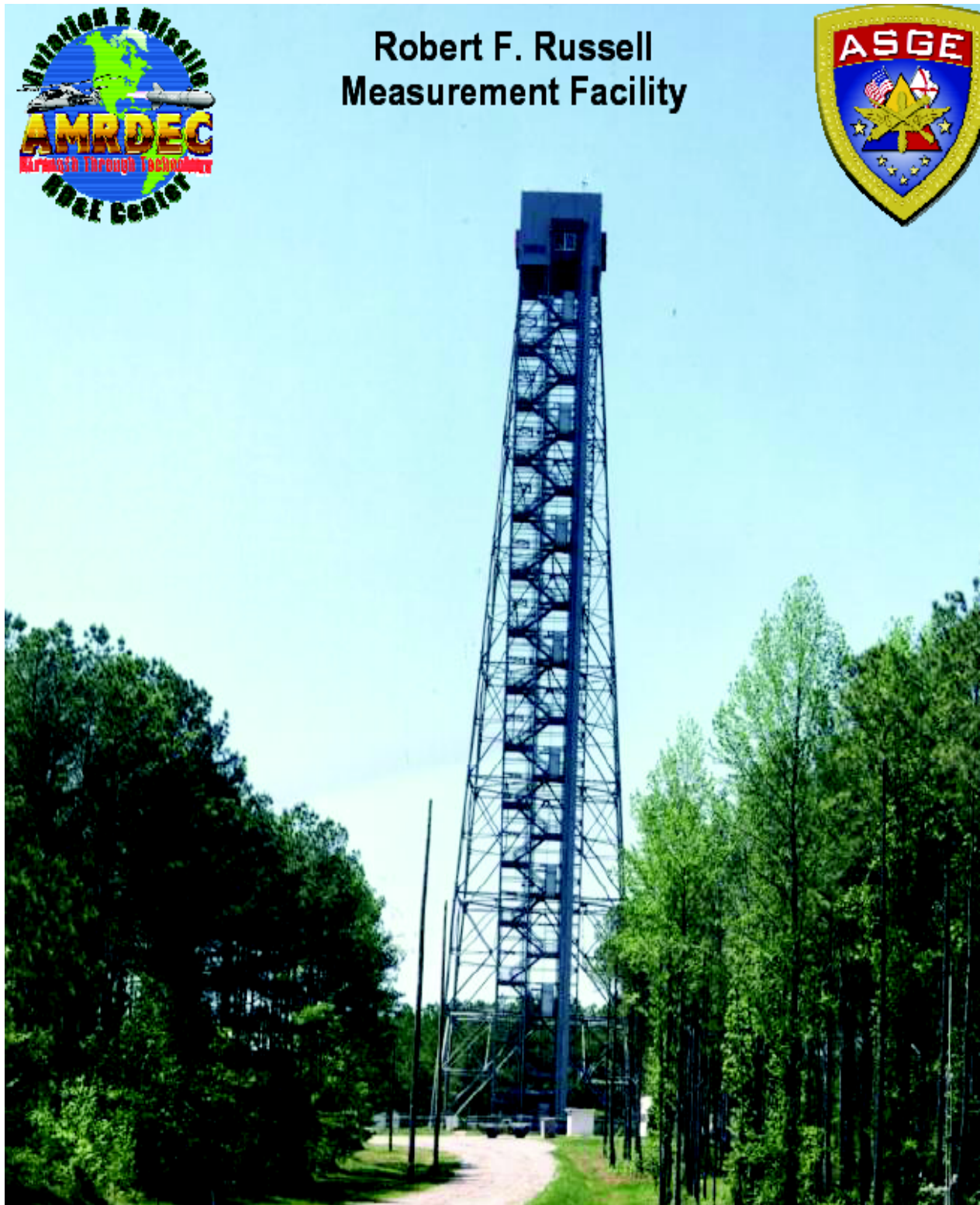
Figure 8: Russell Tower facility @ Redstone Arsenal Alabama.
